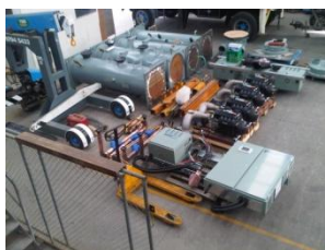
Level 52 chiller strip down
