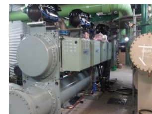
Level 52 chiller in position
