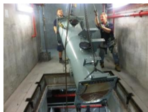
Lifting Level 52 chiller into position
